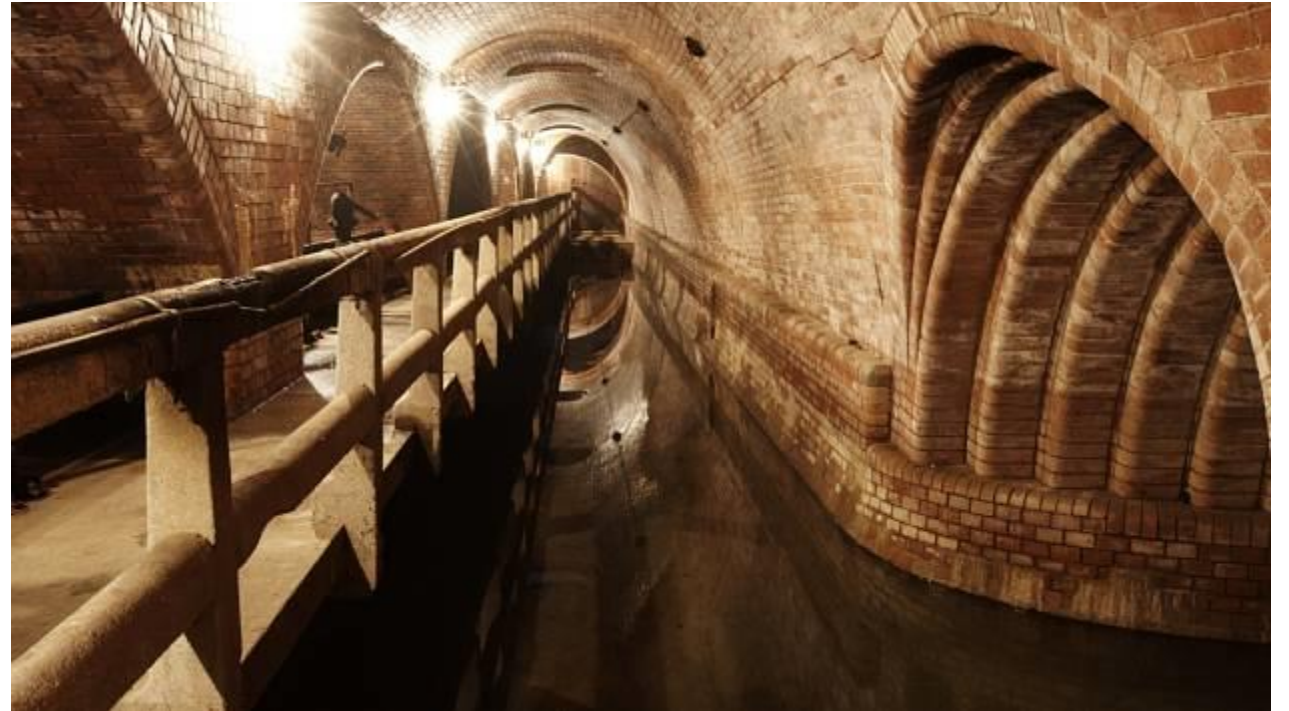
Historical Sewer under Prague
