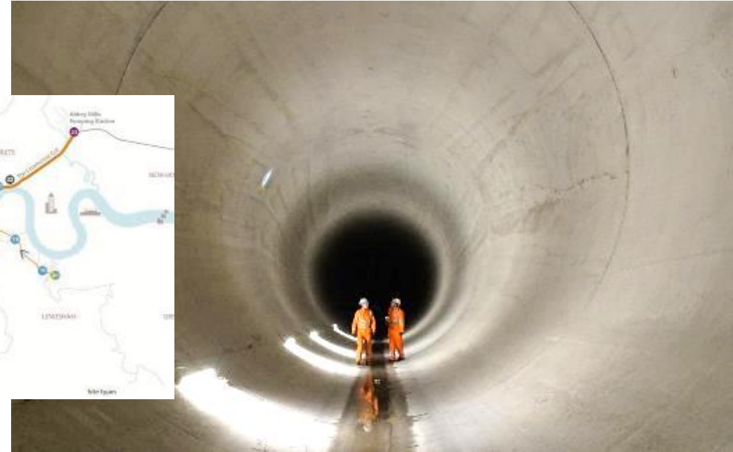
Inside London's £5bn super sewer
