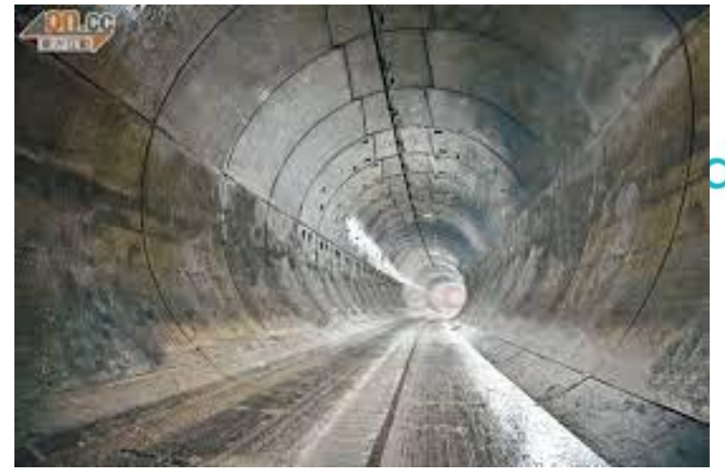
Hong Kong Island Flood Relief Project
